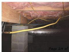
recommend contacting a licensed electrician to verify the piping is properly bonded to the main grounding system as suggested by the pipe manufacturer.
